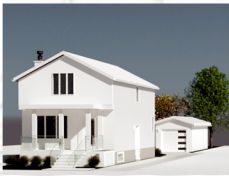
Modern Era House Renovation Toronto, ON
